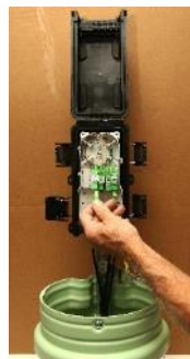
FSDCS4 mounted in an R02 Pedestal
