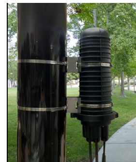
Figure 5 Pole Mounted FODCC
