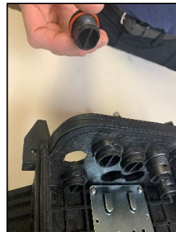
Figure 4 Remove Drop Port Plug
