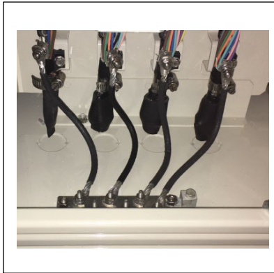
Figure 9 Cable Attachment Hardware Connected to Ground Bar
