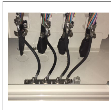
Figure 10 Cable Attachment Hardware Connected to Ground Bar
