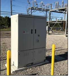
**CUBE Site Support (SS) Cabinet Series** Supports separate chambers for power and, electronics, as well as various battery technologies. May be mounted on Charles CPAD composite material mounting platforms for quick on-site installations.
