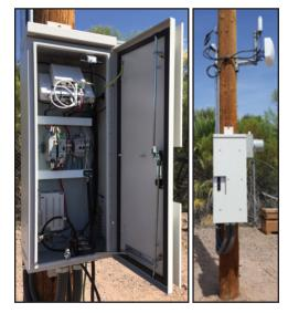
**FAN Remote Cabinets** Mount to utility poles or on the side of a utility box. Serves as a multi-purpose outdoor enclosure for various electronic components and equipment.
