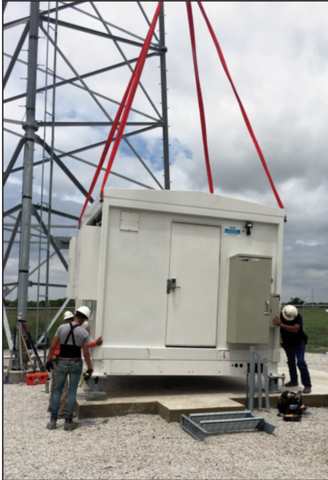
On-Site Crane Installation
