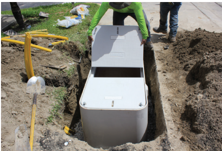
Optional split lid covers facilitate lid removal, access, and technician safety
