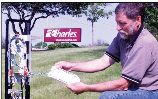
Technician-friendly Charles Fiber Splice Trays are easily removed from pedestal enclosures without disturbing existing splices. A hinged tray is also available.
