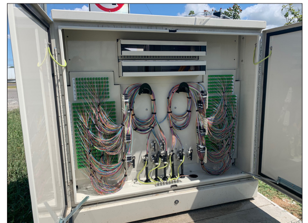
OHC2-864 cable compartment with factory installed pigtails
