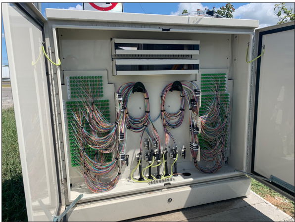
OHC2-864 cable compartment with factory installed pigtails
