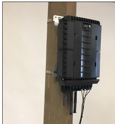
Figure 11 Pole Mounted FSDC
