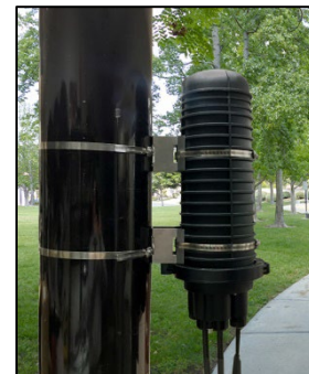
Figure 6 Pole Mounted FODCB
