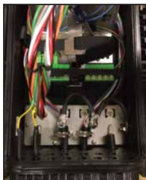
Feed Port, 2 Branch Ports, 16 Drop Ports
