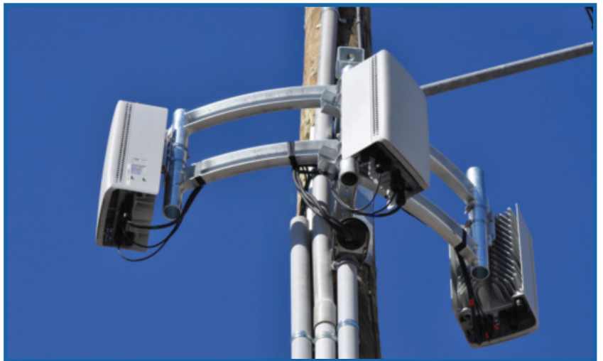
97-5GWDMTHGN1-A installation with (3) customer-supplied 5G radios
