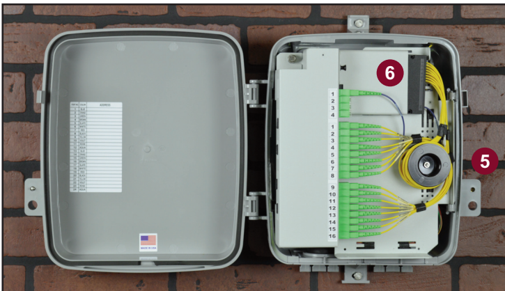
Swing-Out Fiber Bulkhead (Drop Side)
