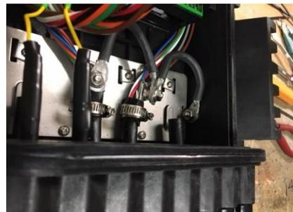
5. When the closure is ready for field installation, attach a customer supplied ground cable to the external side of the ground stud.
