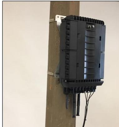
**Figure 11** Pole Mounted FSDC
